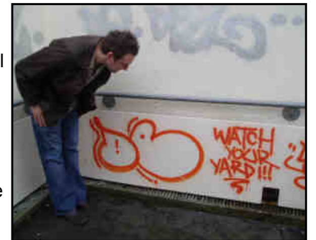
Martin Goss assessing the situation at the Tuffnell Way underpass
